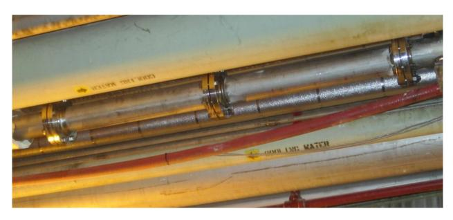
Contaminated and clean 30" [762mm] pipe spool sections
