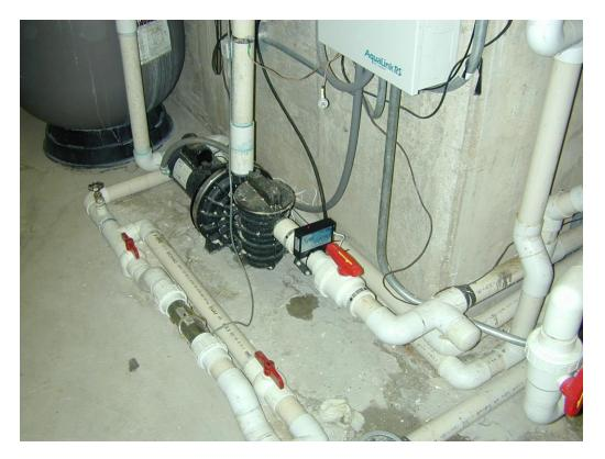
Photograph of installed HydroFLOW water conditioner
